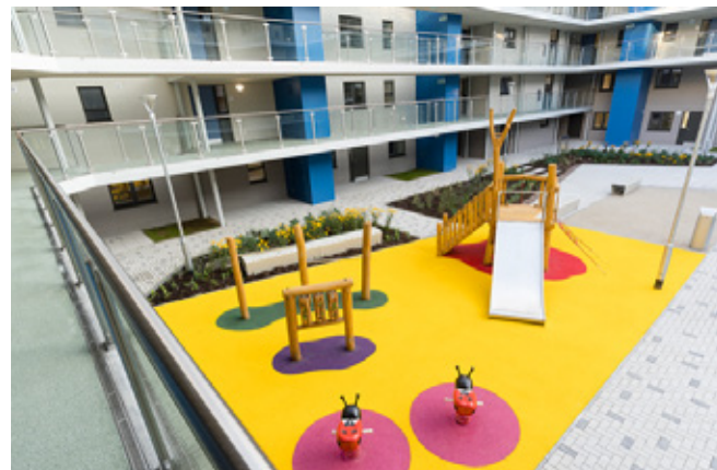
St Marys Mansions redevelopment project, Dublin 1
